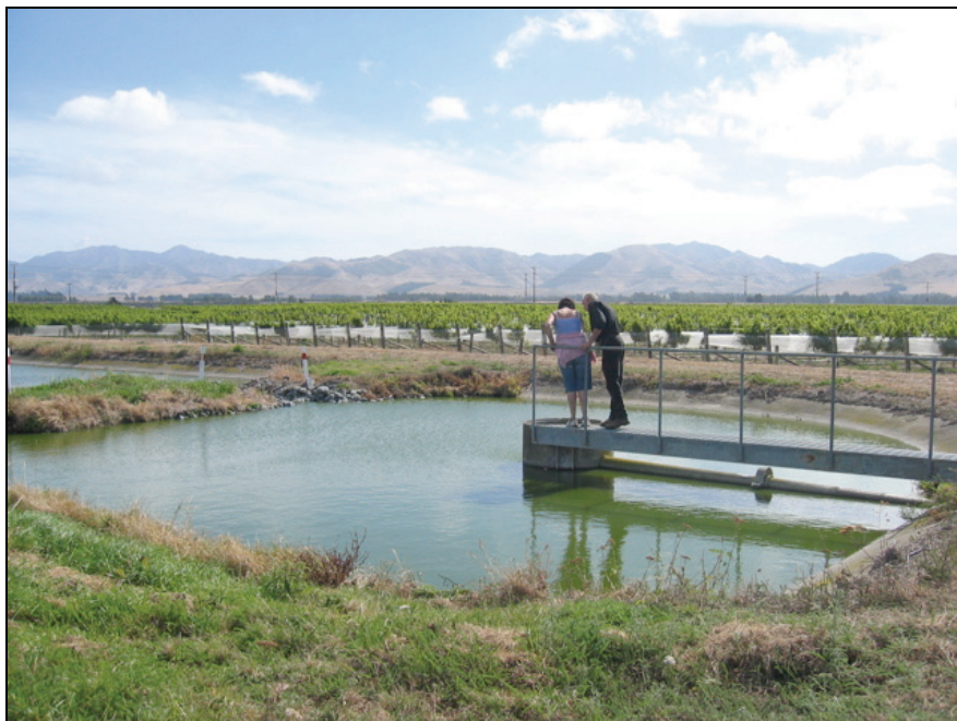
Photo 1: Final oxidation pond, Seddon Sewage Treatment Plant
