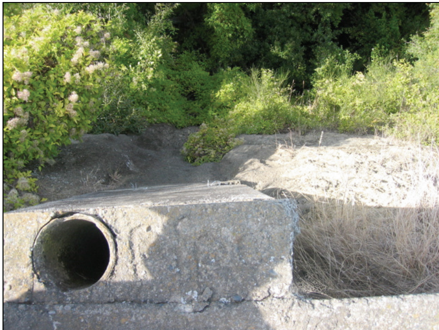
Photo 3: Discharge outfall, on the true left bank of the Starborough Creek
